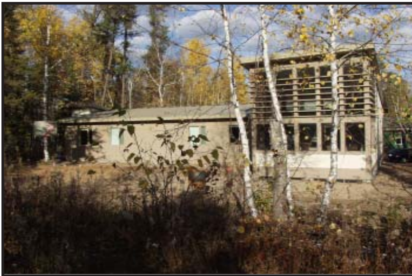
This new, eight-bedroom residence is used primarily by graduate students, and by some of the younger staff spending more than 120 days on site annually. Currently used spring through fall, it is well-insulated and capable of use on a year-round basis.
